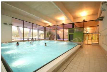
Optimised indoor air humidity reduces heat emission due to evaporation. Photo: PHI
