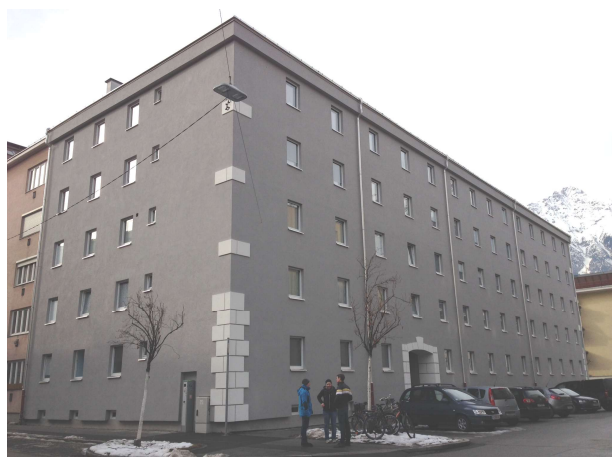
FIGURE 10: VIEW OF THE BUILDING AFTER THE RENOVATION (SOURCE: PHI)
