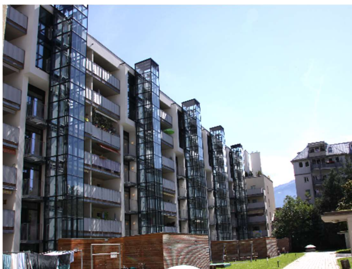
FIGURE 36: VIEW OF THE BUILDING AFTER THE RENOVATION (SOURCE: PHI)
