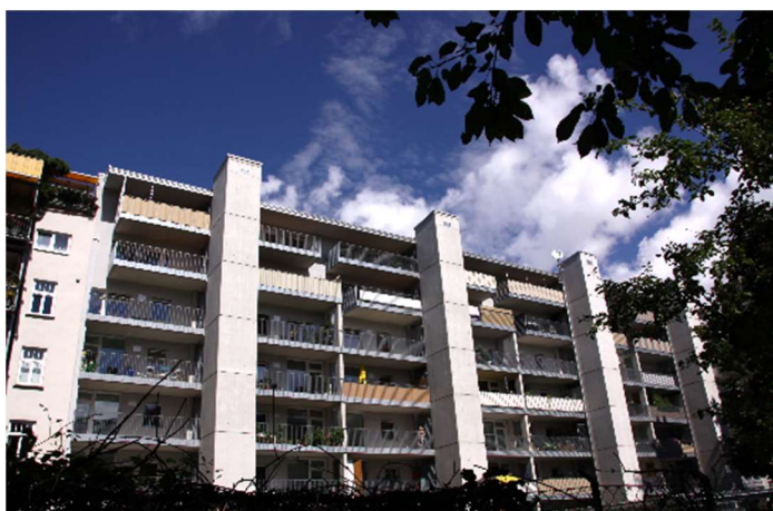
FIGURE 14: VIEW OF THE BUILDING AFTER THE RENOVATION (SOURCE: PHI)
