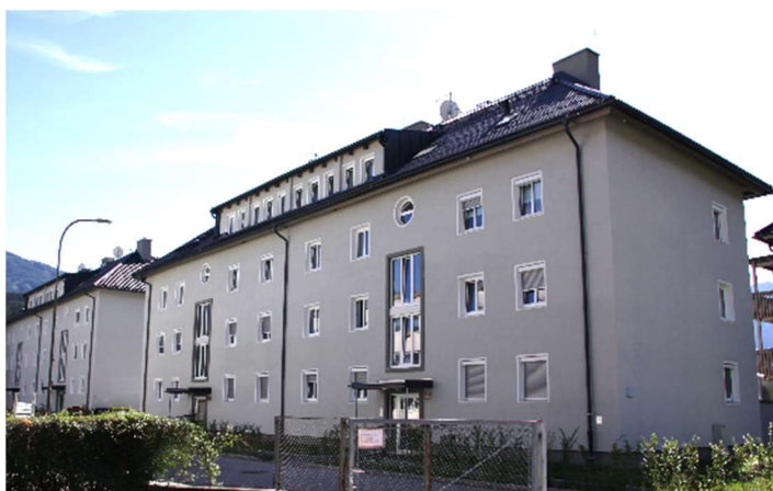
FIGURE 43: VIEW OF THE BUILDING AFTER THE RENOVATION (SOURCE: PHI)
