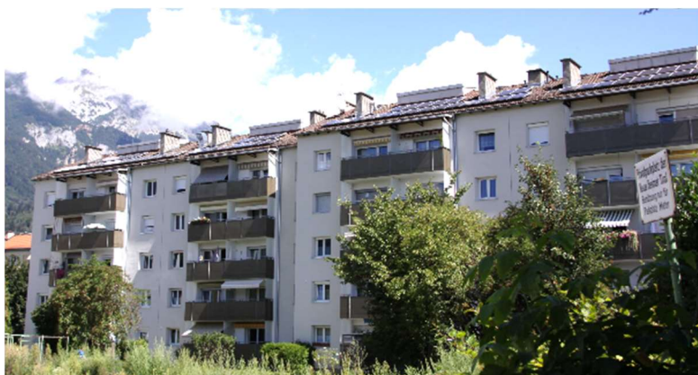
FIGURE 39: VIEW OF THE BUILDING AFTER THE RENOVATION (SOURCE: PHI)
