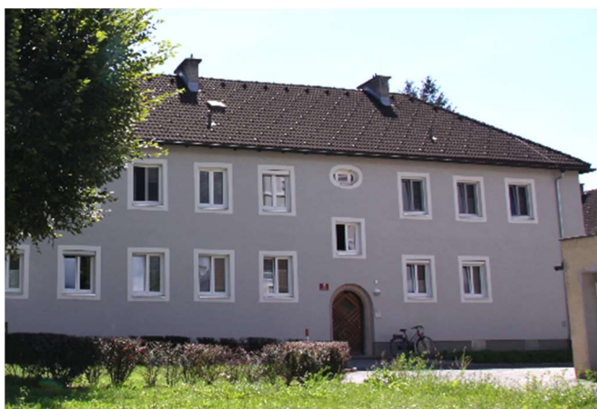
FIGURE 51: VIEW OF THE BUILDING AFTER THE RENOVATION (SOURCE: PHI)
