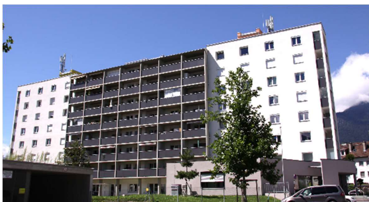
FIGURE 32: VIEW OF THE BUILDING AFTER THE RENOVATION (SOURCE: PHI)
