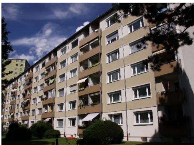
FIGURE 47: VIEW OF THE BUILDING AFTER THE RENOVATION (SOURCE: PHI)
