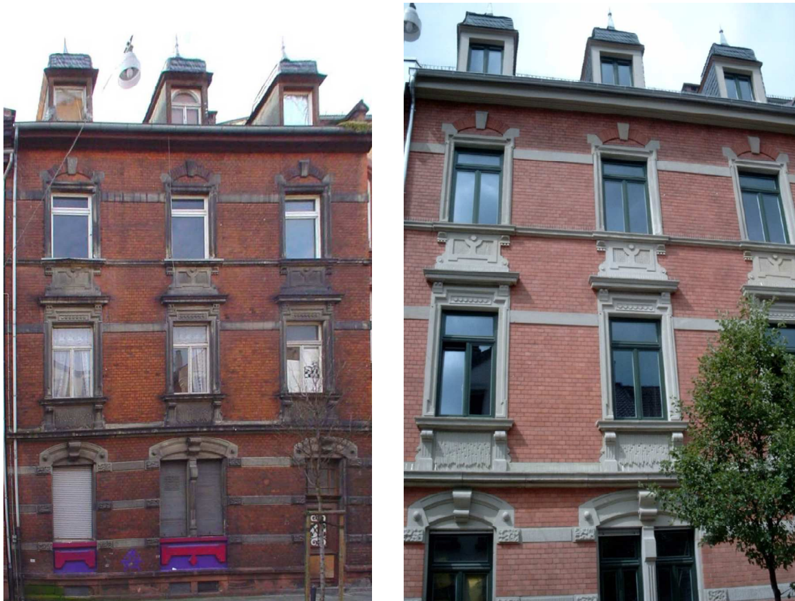
Figure 1: One of the example buildings for the economic assesment: Wilhelminian apartment house in Ludwigshafen, Germany before (left) and after (right) refurbishment (Images: Osika GmbH)
