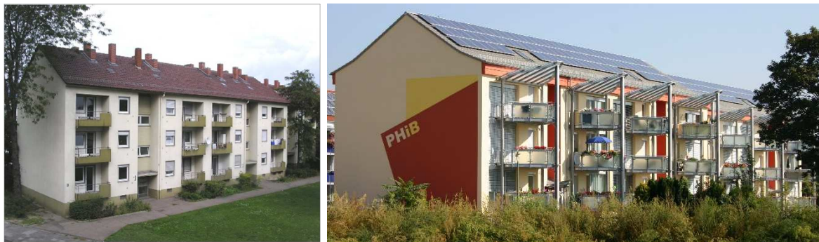
Fig. 15: Building in Hoheloostraße in Ludwigshafen a.R. before and after complete refurbishment. The balcony recesses were used to increase the living space and a balcony system was installed in front.
