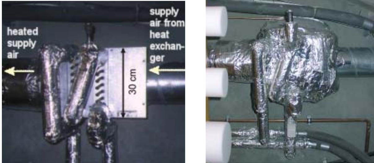
**Figure 22: Postheater in the inflow pipeline (before and after the addition of insulation)**
